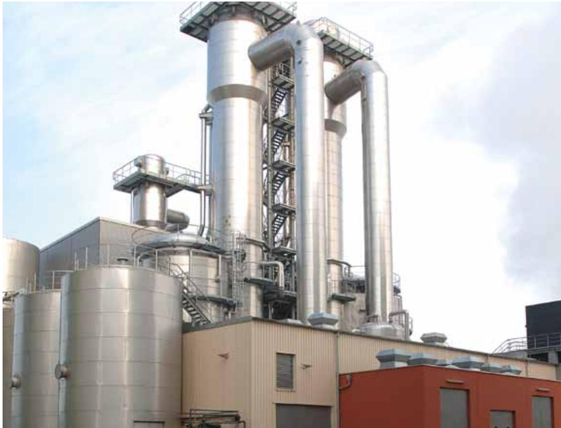
Evaporation plant for the concentration of potato fruit water, consisting of two identical lines; each line with a single-effect falling film evaporator as pre-evaporator, heated by a mechanical vapour recompressor, as well as a 3-effect falling film forced circulation finisher, heated by a thermal vapour recompressor. Overall evaporation rate: 152,000 kg/h.
